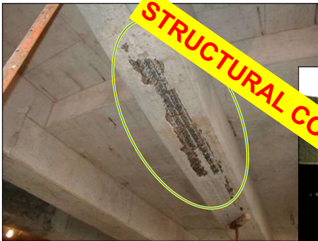
Honeycombed Concrete
