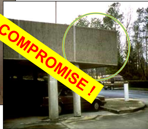
Missing Reinforcement
